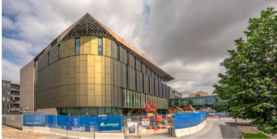
Facade with SolarLab modules, Kromatix coated frontglasses – Module / BIPV-Fassade: SolarLab, Denmark
