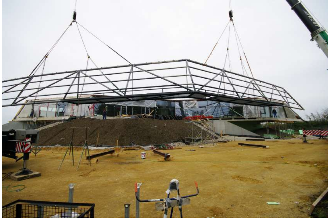
2 mobile crane lift the construction synchron
